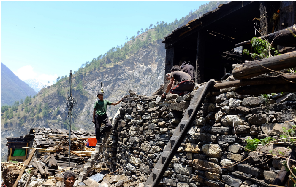
Figure 1. House under reconstruction shortly after the first major earthquake.
