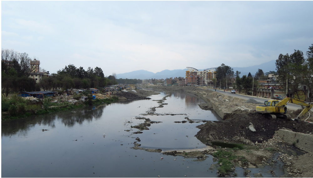
Figure 1. Concrete embankments and roads built along the Bagmati River.
