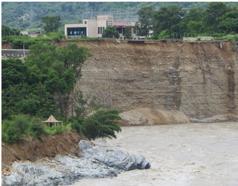
Figure 4: Erosion of muck disposal site at Srinagar Dam, after the flood of June 2013.
