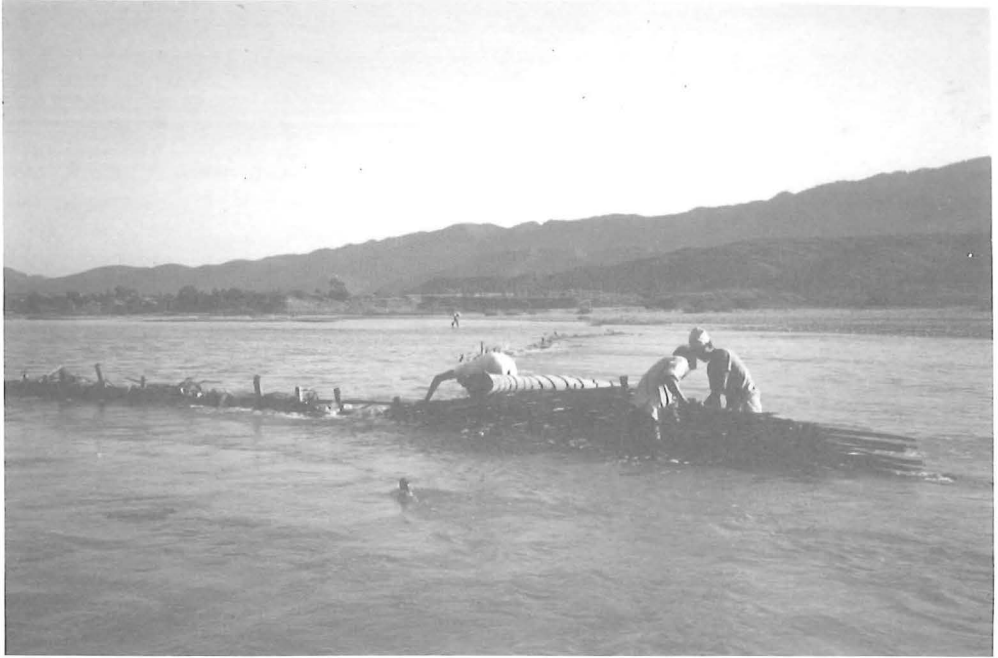
Photo 5 : A large tip dam in the Babai river in Dang. Men are fixing the conical trap.
