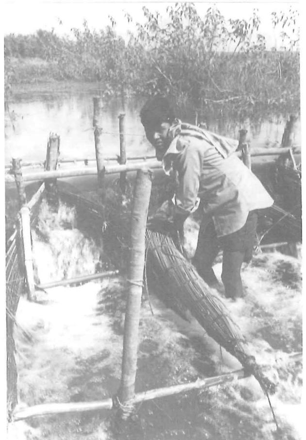
Photo 7 : Fixing a conical trap on a small dam.
