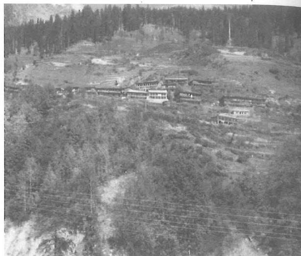
Figure 4 Solang Village viewed from across the river
