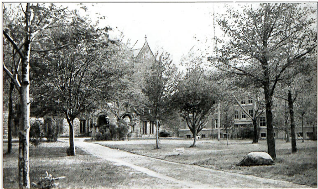
APPROACH TO MAIN BUILDING AND SCIENCE HALL
