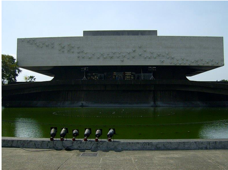
Figure 4. The Main Building of the Cultural Center of the Philippines. Photo taken by Michael Francis McCarthy.
