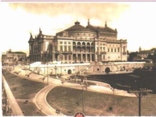
Figure 2.1 Construction of Theatro Municipal de São Paulo
