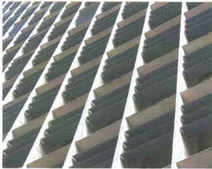
Figure 3.2 An example of brise soleils as seen on the Edificio Copan, 1957
