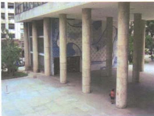
Figure 3.1 An example of pilotis as used on the Ministry of Education and Health, Rio de Janeiro, 1936
