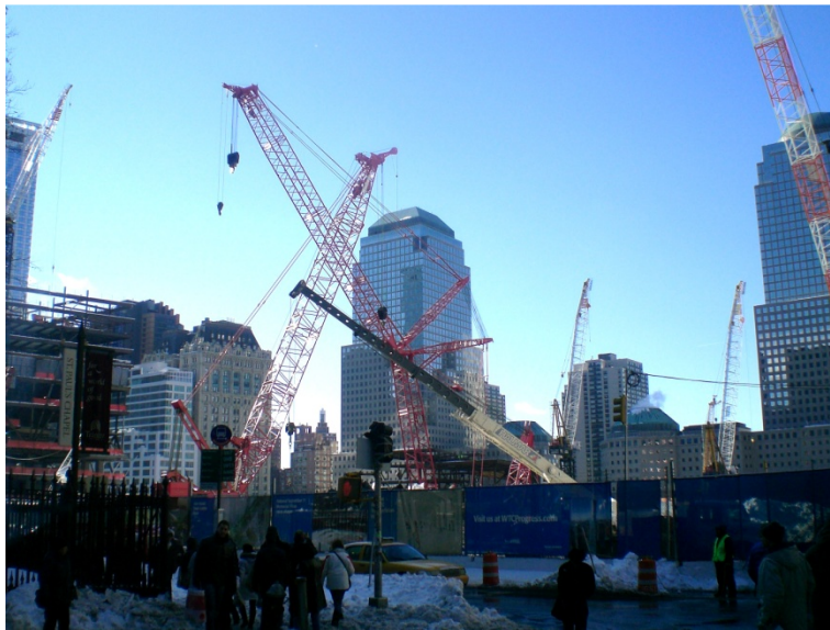
Figure 2: view of the Ground Zero construction site from Church and Vesey.
