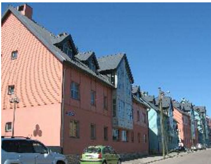
Image 6: New upper-middle class housing built by the Italian firm Breatoni.
