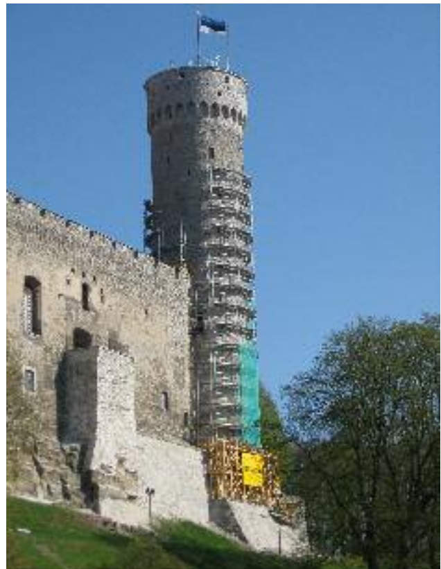
Image 2: Renovations on Toompea Castle, May 2006.
