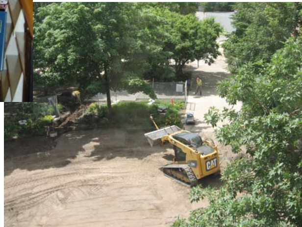
CONSTRUCTION OF MARVIN PLAZA
